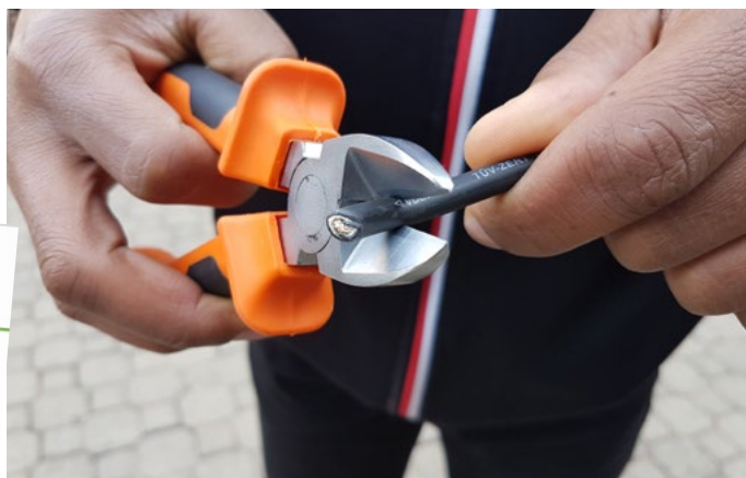
Assist the installer with the joining of solar modules
