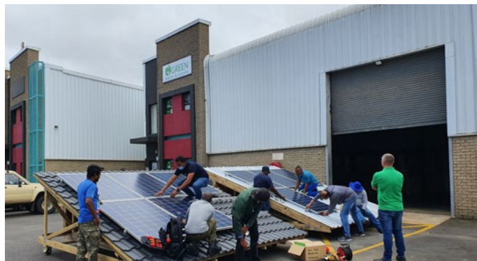
Practical installation day
