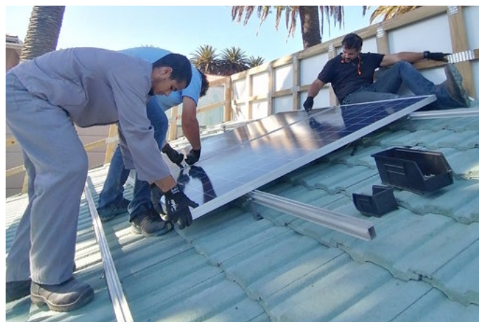
Work practically with solar equipment
