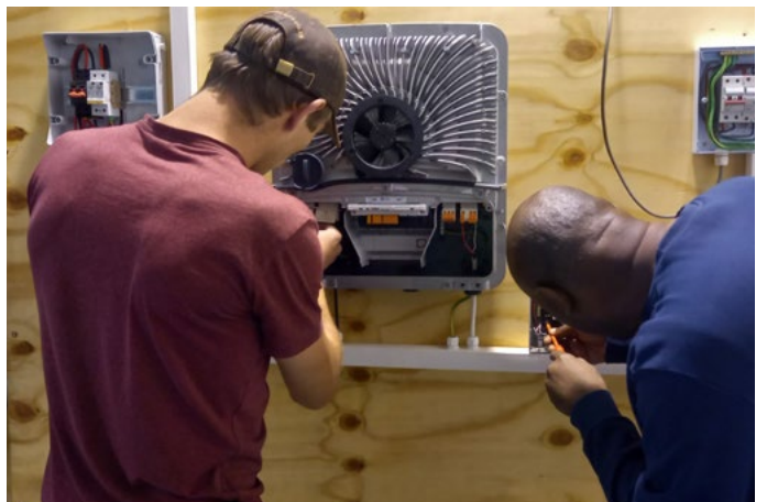
Learning how to connect a PV inverter
