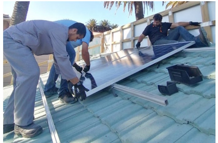
Work practically with solar equipment
