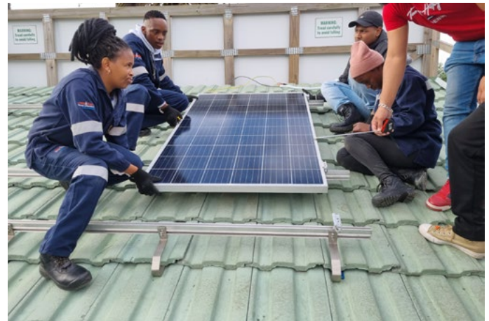
Working practically with solar equipment
