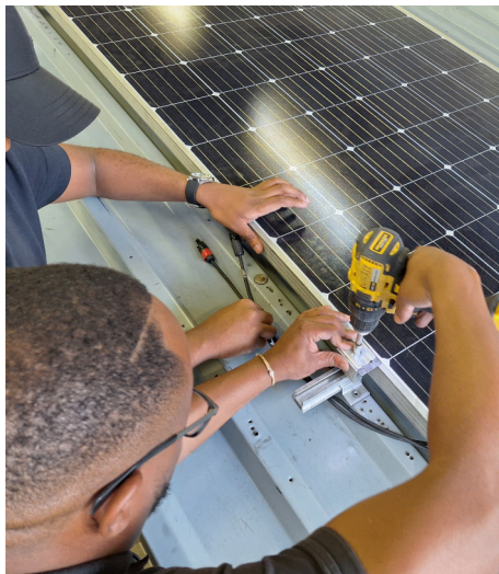
Hands-on training for PV installers
